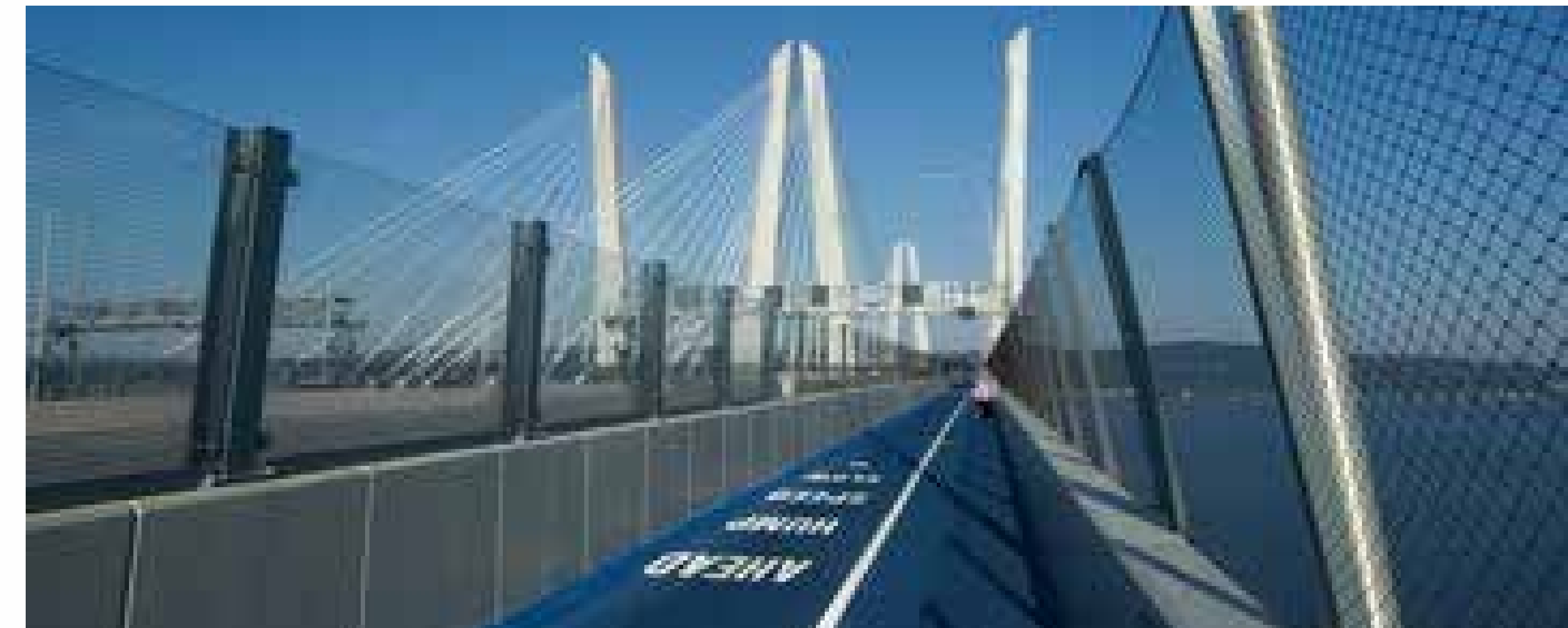
Mario Cuomo (Tappan Zee) Bridge (NY)
