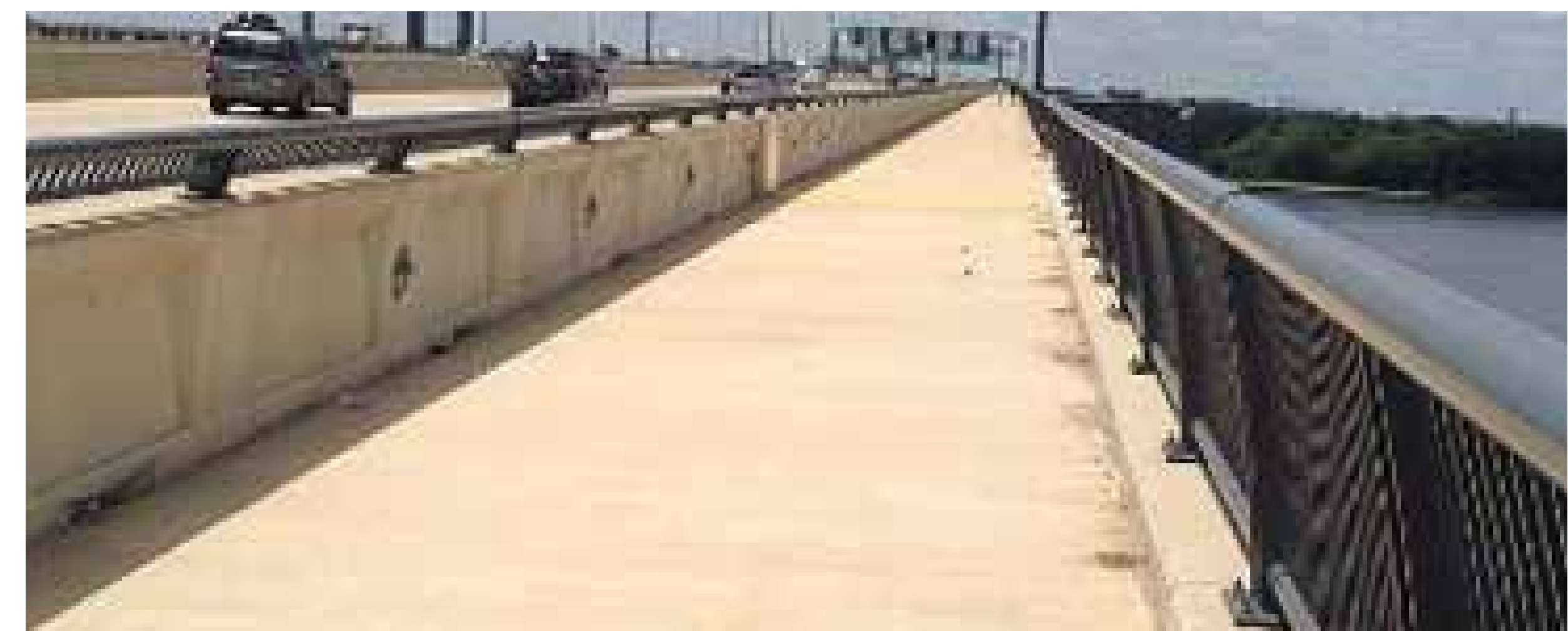
Woodrow Wilson Memorial Bridge (MD)
